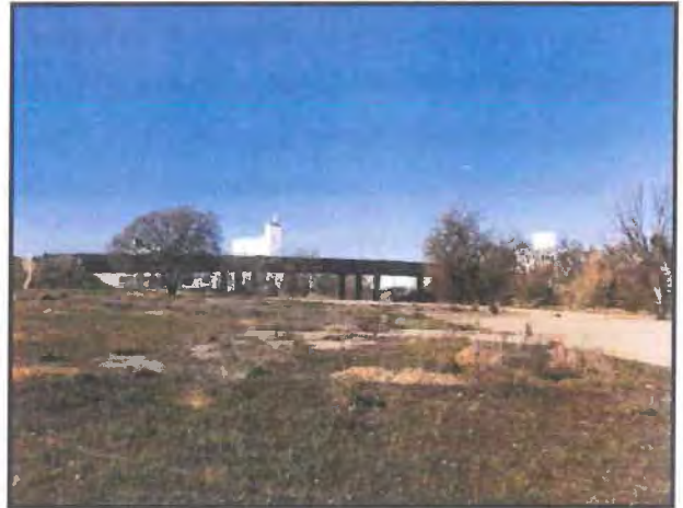
View of Palamidessi Bridge from APN 067-180-036
