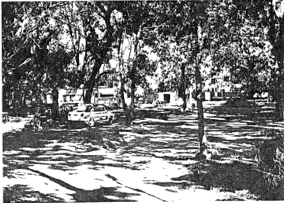
VIEW LOOKING SOUTHEASTERLY FROM BASE OF LEVEE
