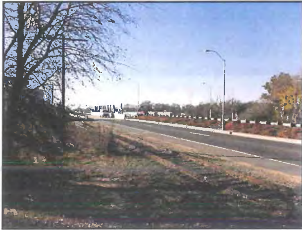
Looking south along Jefferson Boulevard at Bascule Bridge
