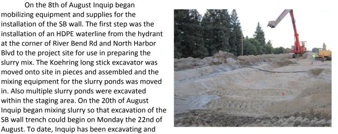
backfilling the SB wall for an entire six day work week. Work began at the east end of the where the SB wall is only 25' in depth. More than 1500' of SB wall trench has been excavated and over 1000' has been backfilled with slurry, and two temporary wall settlement monuments have been installed.
