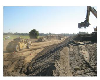
the sandy material was retained and stockpiled adjacent to where the Soil Bentonite wall is to be
