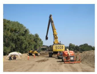
different excavator which was assembled the following day and resumed the excavation on the following Monday, the 19th. To date the slurry wall has been excavated to Station 22+50 leaving less than 500' remaining. The backfill top out is just beyond Station 28+50 and the wall has been capped to Station 29+00. The contractor expects work to be completed by the 1st of October on the Slurry wall and is proceeding with night work beginning Monday the 26th.
